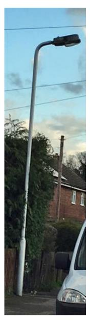
This is likely to be a SON light source so no immediate problems, but this type of lantern is made from a plastic/poly type body which will have been subject to UV degradation so will at some point need to be replaced. I would not say this is an urgent problem, but may be looked at on a point for point replacement.
