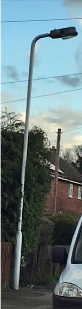
This is likely to be a SON light source so no immediate problems, but this type of lantern is made from a plastic/poly type body which will have been subject to UV degradation so will at some point need to be replaced. I would not say this is an urgent problem, but may be looked at on a point for point replacement.
