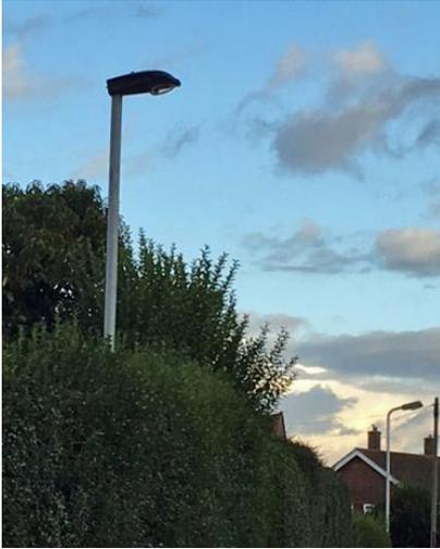
These are fairly modern fittings, and I predict they will be either SON light source or Cosmo already, both light sources are still readily available for lamp and gear replacements. The lantern is also made from a robust aluminium so will have a number of years left of use, the body of these lanterns is expected to last in excess of 15 years (Subject to not being vandalised).
